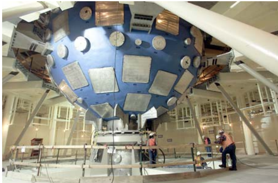
Figure 11 Installation of the “target chamber” at the NIF Inertial Confinement Fusion facility (Source NIF (CNS 2009)).
