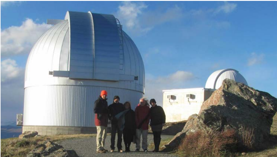
Figure 9. Telescopes used by the MOA collaboration at the University of Canterbury Mt John Observatory in New Zealand. The nearer one has an aperture of 1.8 m, the more distant one 0.6 m. NZ astronomers Nicholas Rattenbury, Grant Christie, Marilyn Head, Warwick Kissling and Jennie McCormick are also shown. A ‘typical’ planet detection by gravitational microlensing is shown in Figure 10.
