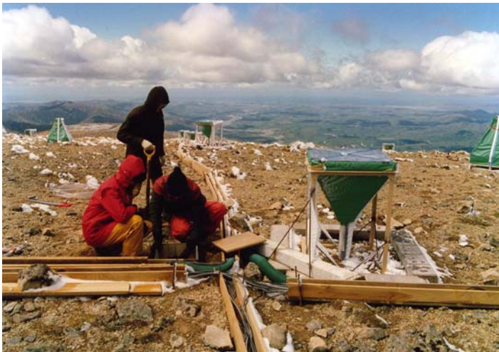
Figure 6. MSc students David Hirst, Peter Norris and Mark Conway of the University of Auckland installing cabling for the JANZOS cosmic ray detector at Black Birch in Marlborough during the winter of 1987. The detector consisted of an array of 76 plastic scintillators that were sensitive to cosmic rays with energies 10^{14} eV to 10^{15} eV, three Cerenkov telescopes that were sensitive from 10^{12} eV to 10^{13} eV, and a central electronics hut. The entire detector covering 5 hectares is shown at Yock (2012).
